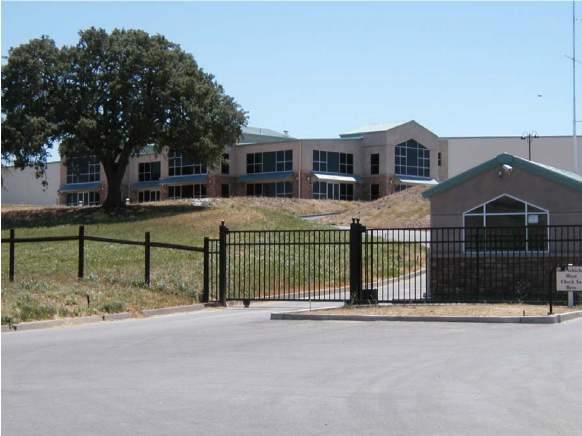
View from front gate
